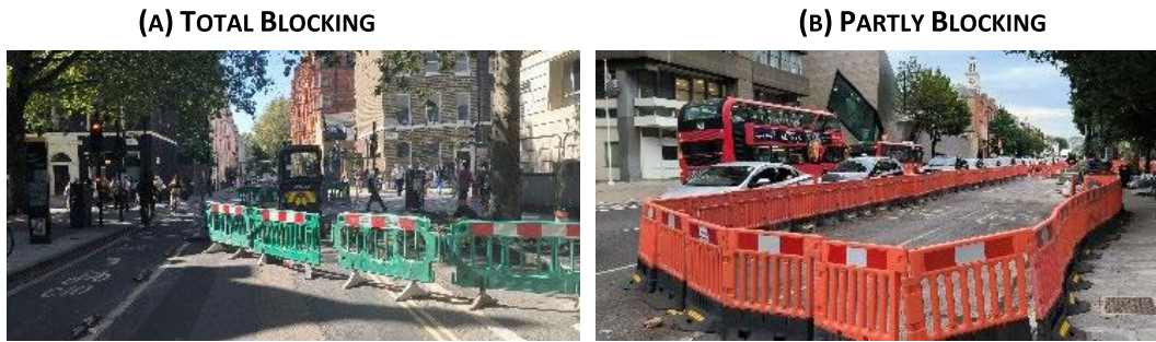
FIGURE 24 ROADS OUT OF SERVICE
