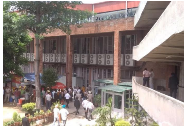
Figure 23: Chaos behind the High Court Building Source: Chandigarh Master Plan 2031
