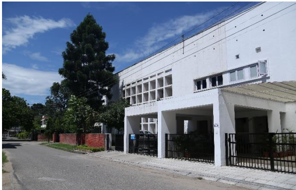
Figure 24: Government housing built by the administration to house government officials in sector 22 (Phase I) Source: Author
