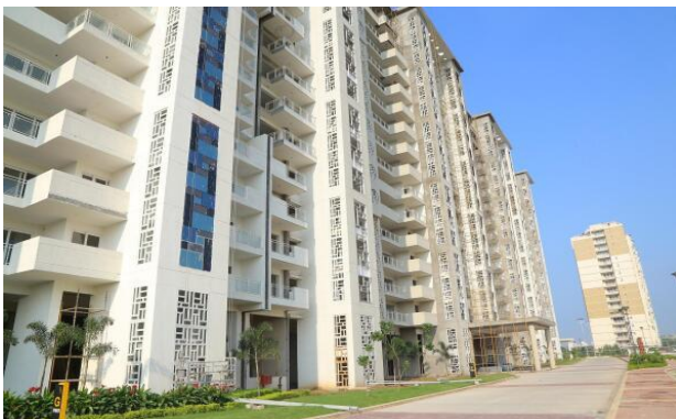
Figure 34: Private high-rise housing in Mohali sector 66A (Present) Source: Author
