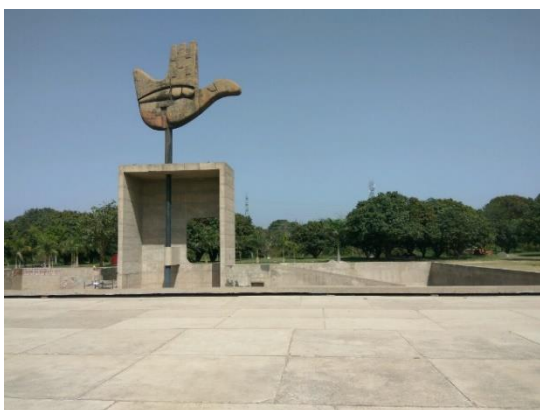
Figure 17: Open-Hand Monument Source: Chandigarh Administration website
