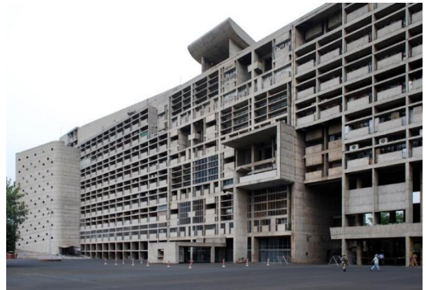
Figure 21: Secretariat building for government of Haryana in Capitol complex; Source: Google Images
