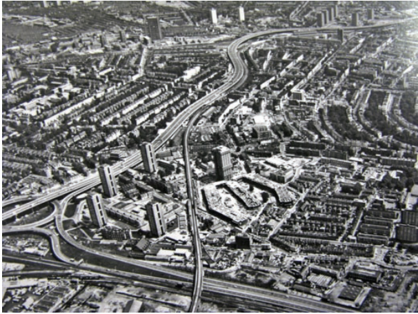
Figure 2. 1973 Aerial view. Source: grasart.com . ©RBKC Local Studies and Archives.
