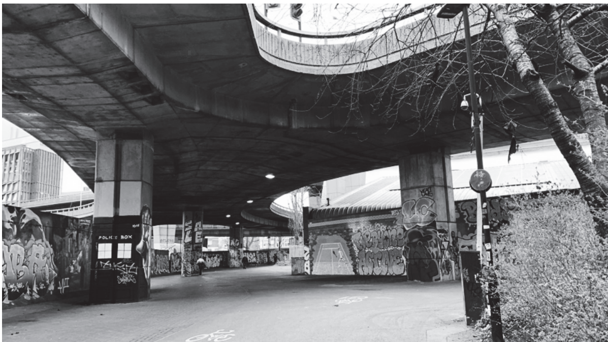
Figure 1. Residual space underneath the Westway, London.
