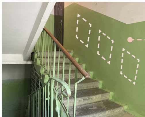
F27. Entrance staircase.
