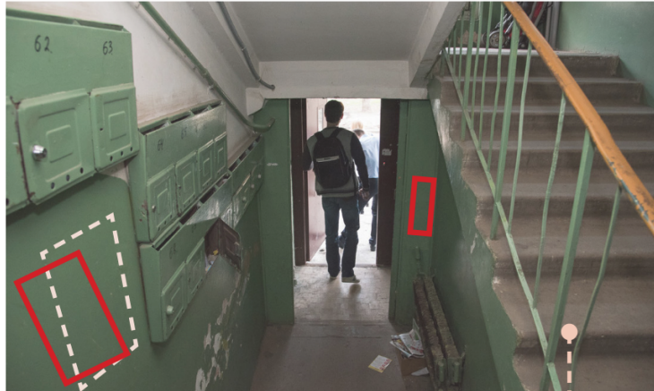
F25. Entrance hallway.
