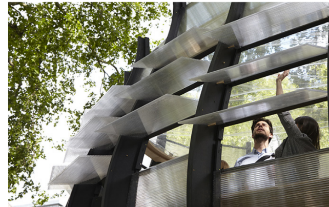
Figure 21: The tree-house received natural light through the transparent plastic (Urban Design Mag, 2015)
