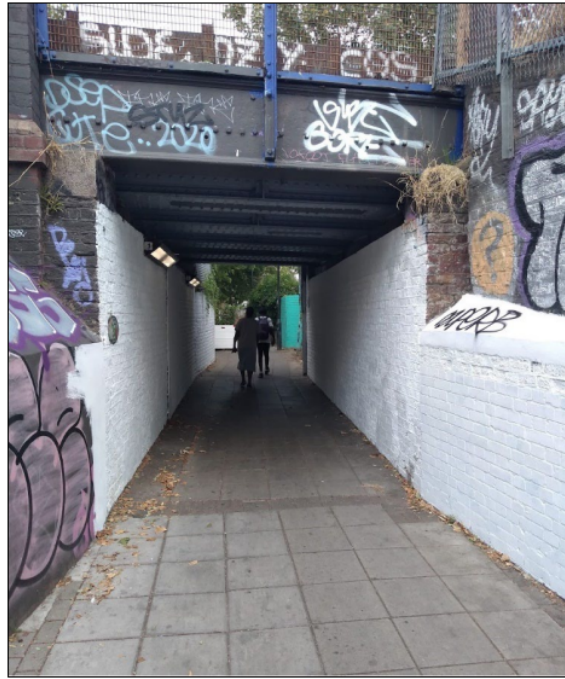
Figure 47 – Fresh re-painting of the Somerleyton Passage underpass (Author's own,2022)
