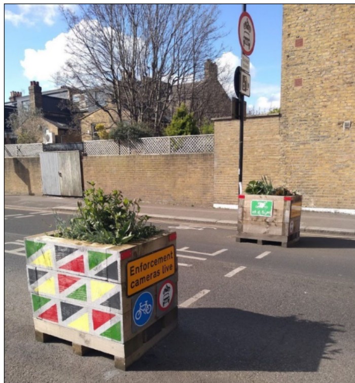
Figure 45 – Council modal filters by besides Kellett Road within the Railton LTN (Author's own,2022)
