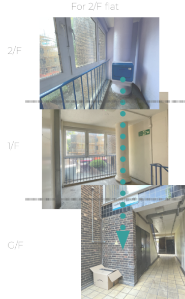
Existing public housing - Chute system
