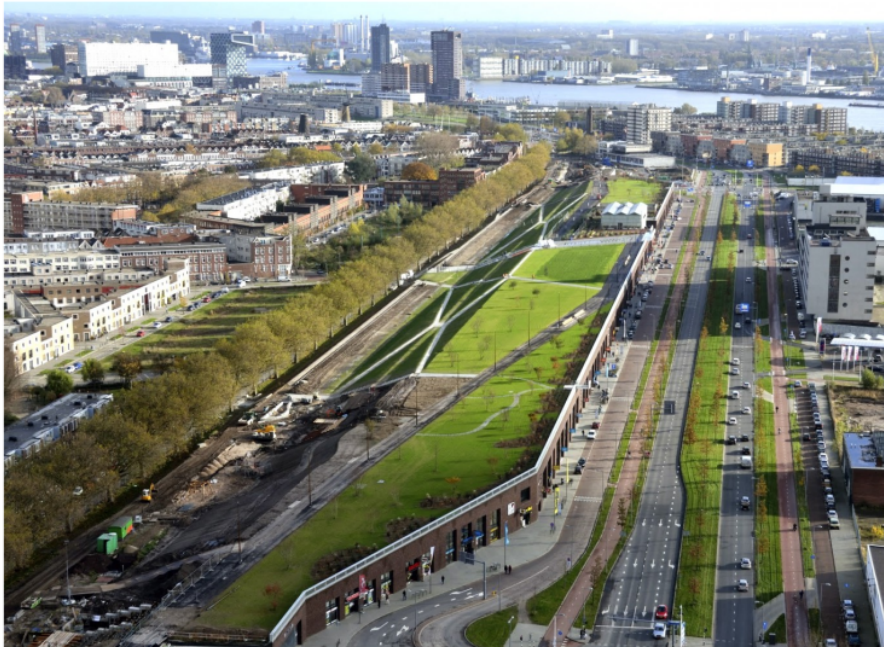
Under construction. Source – Buro Sant en Co
