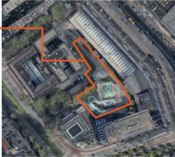
Watersquare Bentemplein Location: Agniesebuurt, Rotterdam North – outer city centre/residential area fringe Area: 9000m 2
