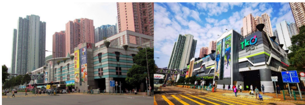
Figure 9: TKO Spot before and after refurbishment (Link, 2022)
