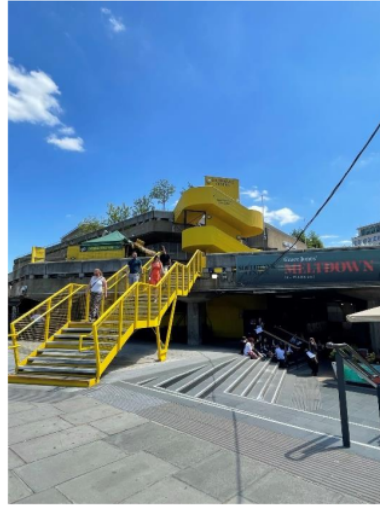
Photo 7 - Multi-level: The public space around South Bank Centre has several different levels connected by stairs, painted in bright yellow that contrasts well with the rest of the bare concrete. This helps able-bodied users identify connections between levels, but also makes it difficult for those who can't use stairs to find accessible options.
