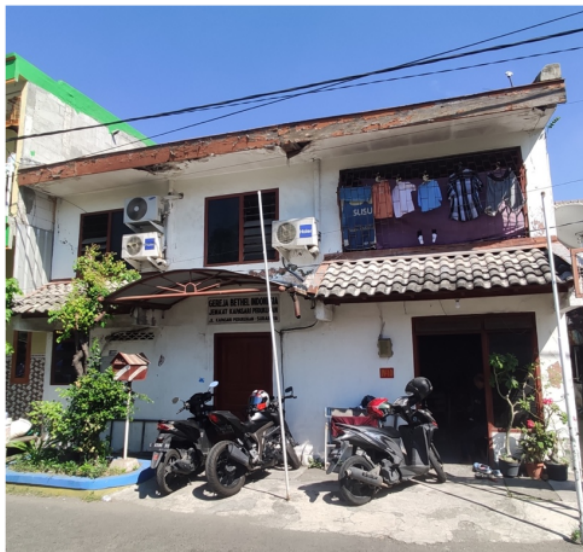
Figure 53. G5 - house facade
