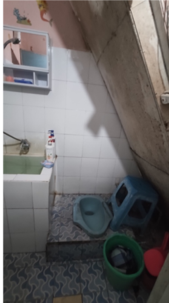
Figure 56. G5 – bathroom 1 st floor
