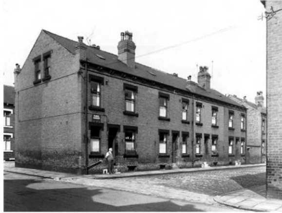
Figure 21. Back-to-back terraced housing in Leeds (source: Leodis.net)
