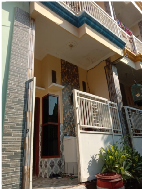
Figure 40. G3 - house facade
