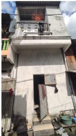
Figure 49. G4 – house facade
