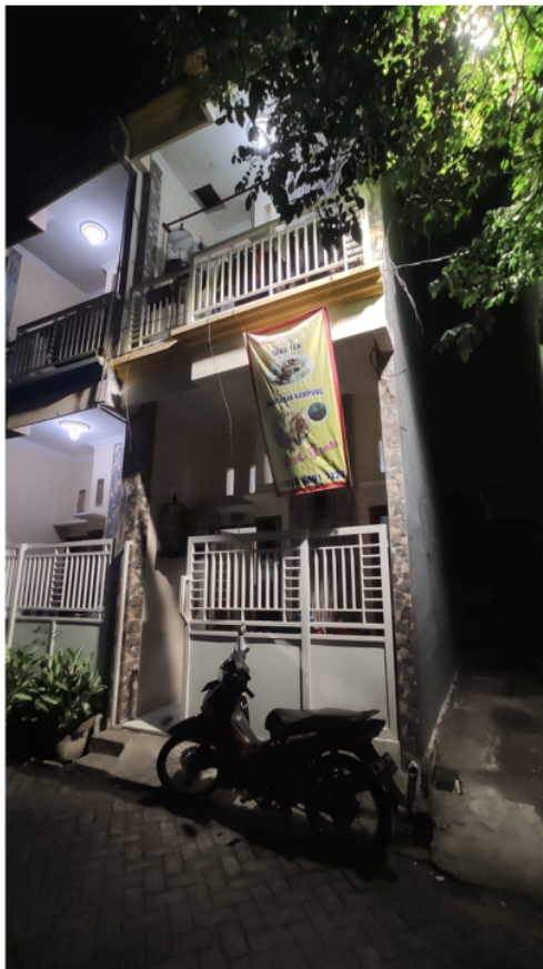
Figure 32. G2 – house facade
