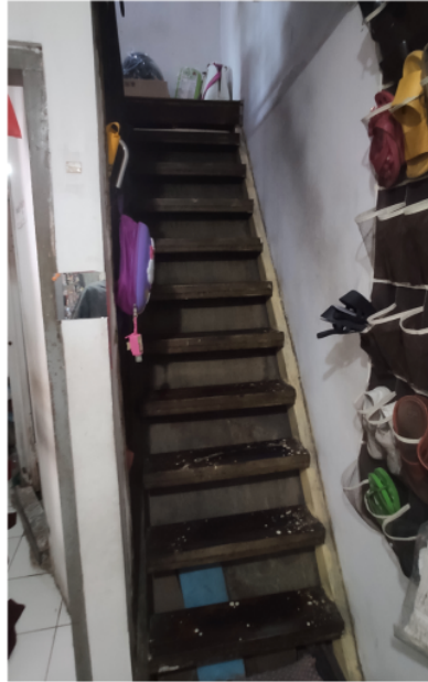
Figure 20. Stairs in G5 house.
