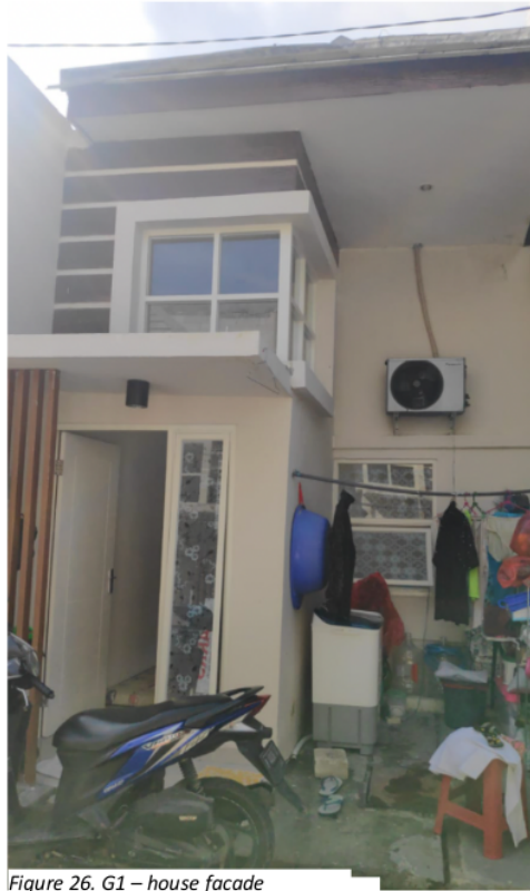
Figure 26. G1 – house facade
