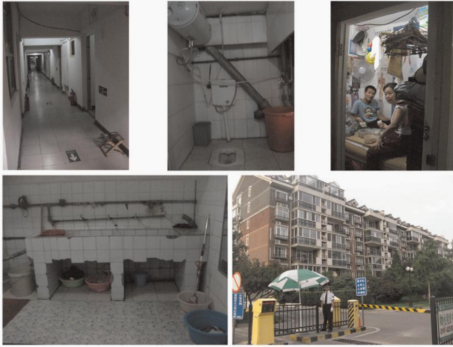
Figure 10: Basement condition, and above-ground apartments (source: Huang and Yi, 2015).
