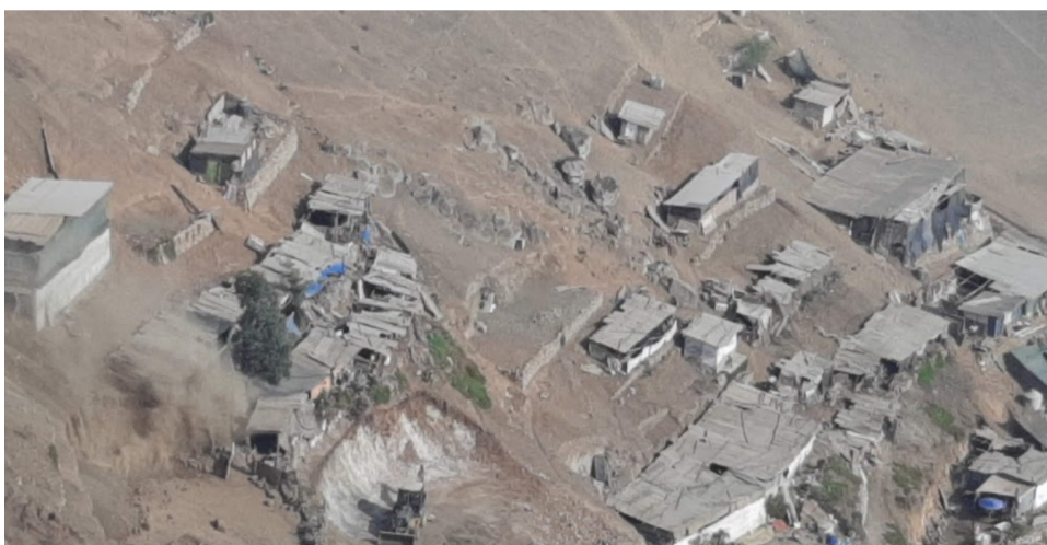
Figure 11: Highest point of Villa Maria del Triunfo at 400m above sea level (Google maps, 2021)
