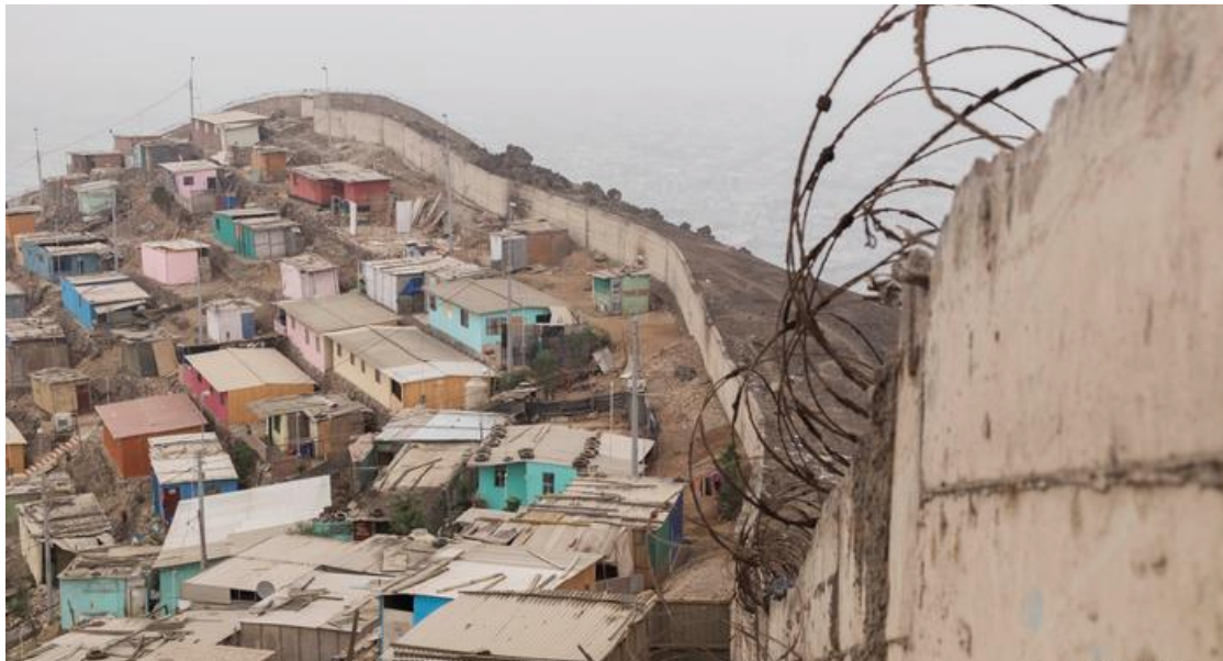
Figure 6: The wall dividing Villa Maria del Triunfo and La Molina (Van Eertern, 2017)
