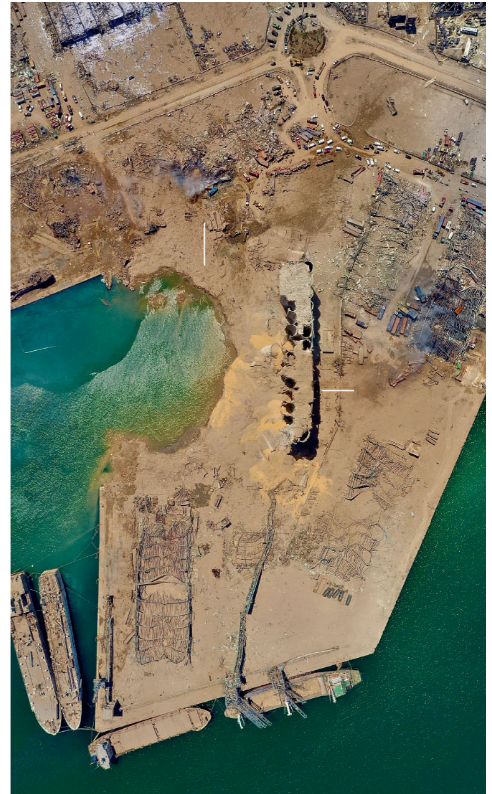
Figure 001: Satellite Image of Port Damage (2020) (Source: New York Times)
