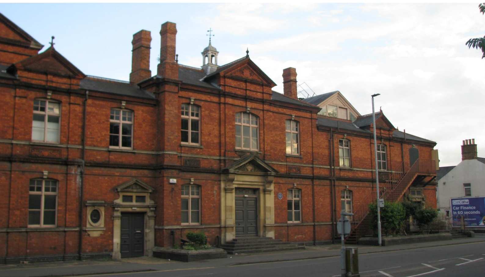
Fig. 34 (Below) the GWR Swimming Baths and Dispensary's Northern Façade.
