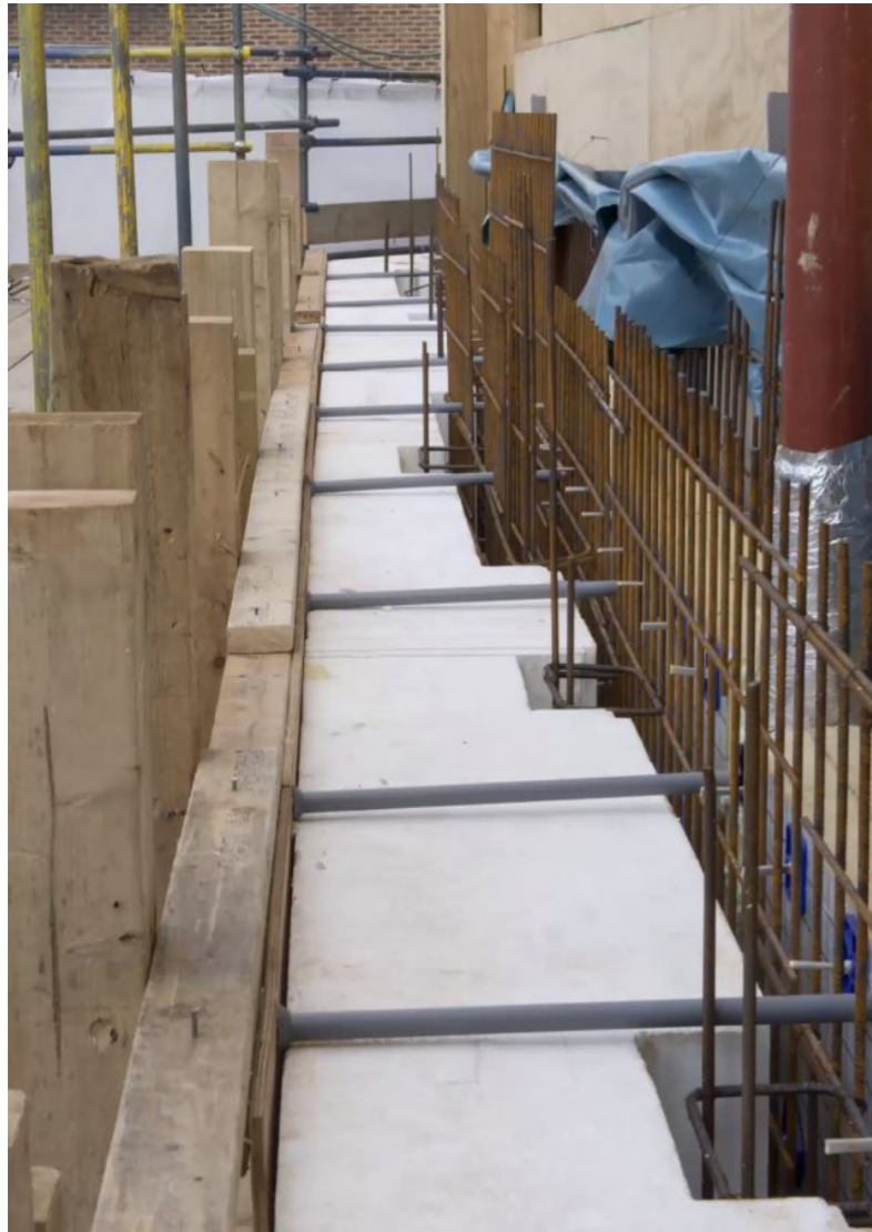
Fig. C09 (left): Polystyrene mould wall before casting Aria building.
