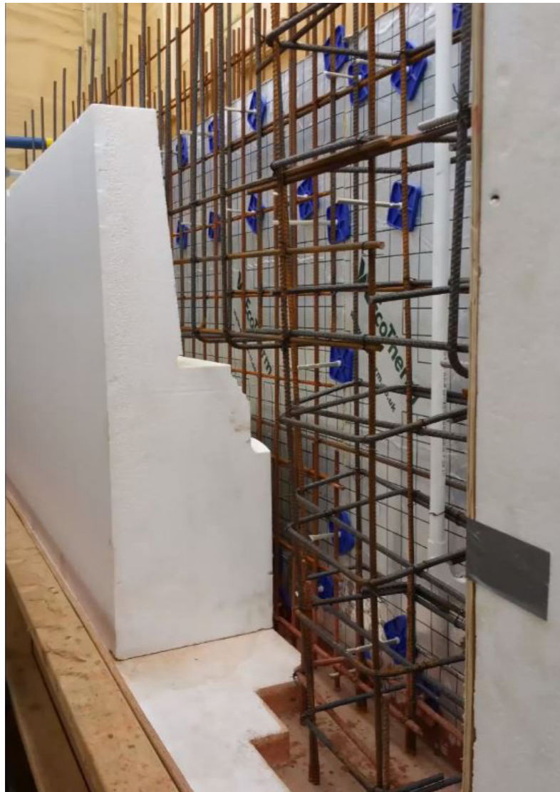
Fig. Po3 (left): The polystyrene mould construction method could be use for the plaster workshops.
