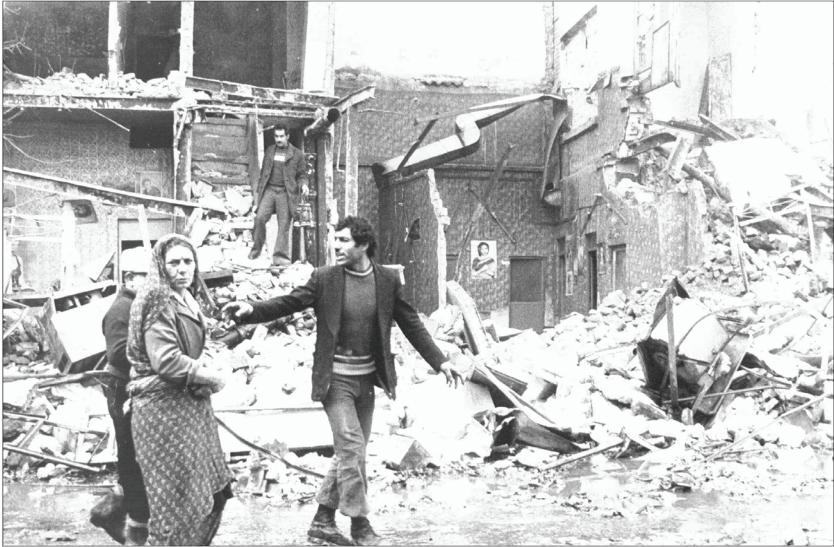
Figure 6: A demolished brothel in Shahrinaw, 1980, photographer Unknown, National Library and Archive of I. R. Iran
