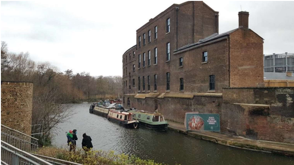
Figure 57. Regent’s Canal in King’s Cross, London (Source: Author’s photographs)
