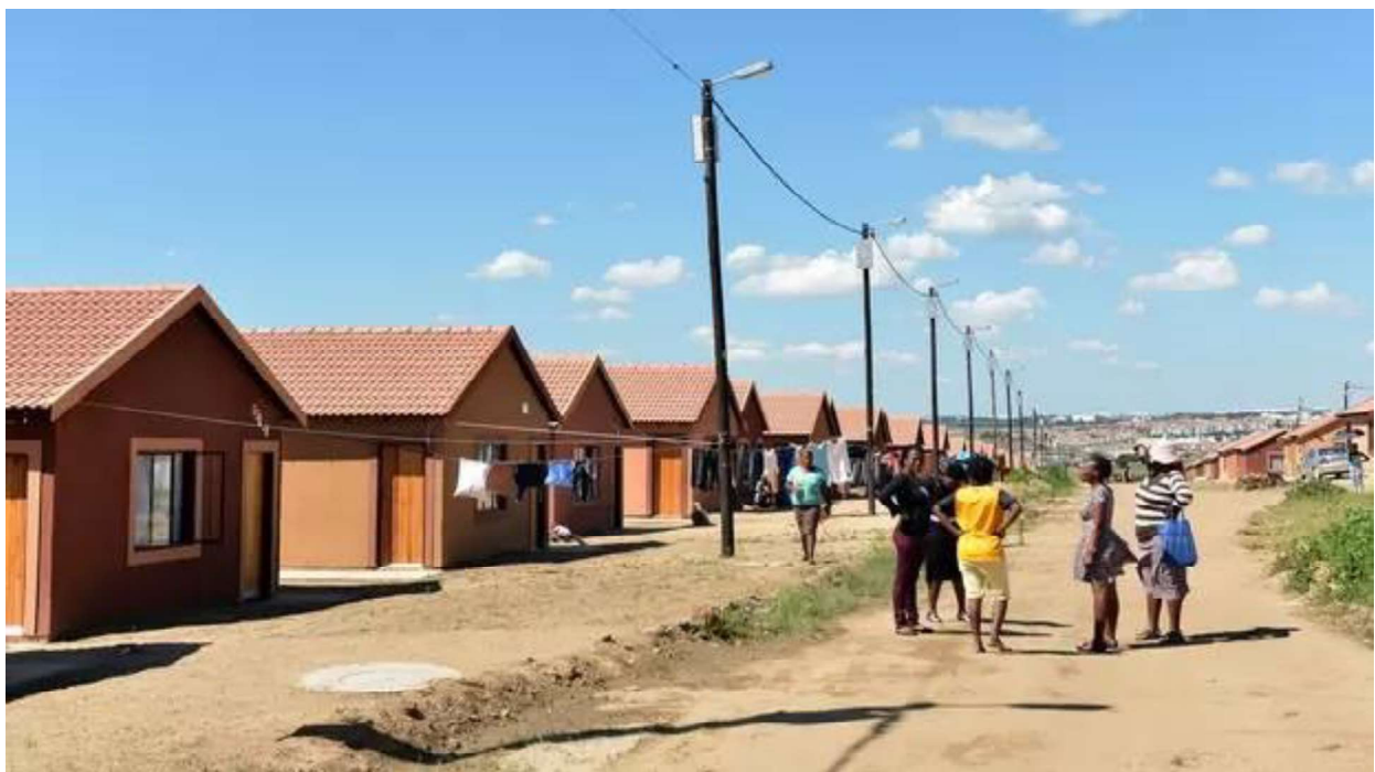
Figure 9: Example of RDP Houses in South Africa
