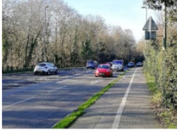
Fig. 10. Segregated shared pavement. Woking, Surrey. Source: author.
