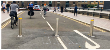
a) South-East Entrance
