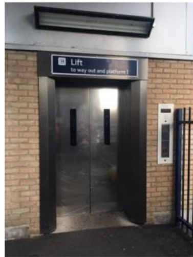
Figure 5 Lift at an Accessible Station
