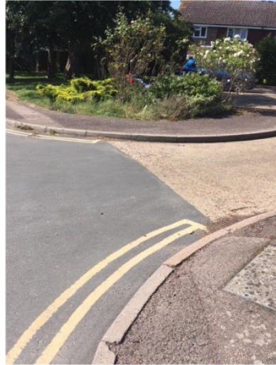
Figure 3 No Dropped kerbs at Crossing
