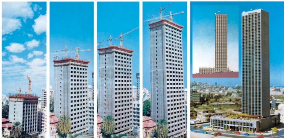
El Murr Tower was built in the 1970s, and was the highest tower of its time, the 40-story building was built at a pace of one floor every day. El Murr Tower is located in the heart of Beirut and incorporates modern apartments and offices.
