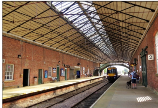
Figure 6 The splendid hipped timber and glass canopy of Grade II* Listed Filey station, North Yorkshire
