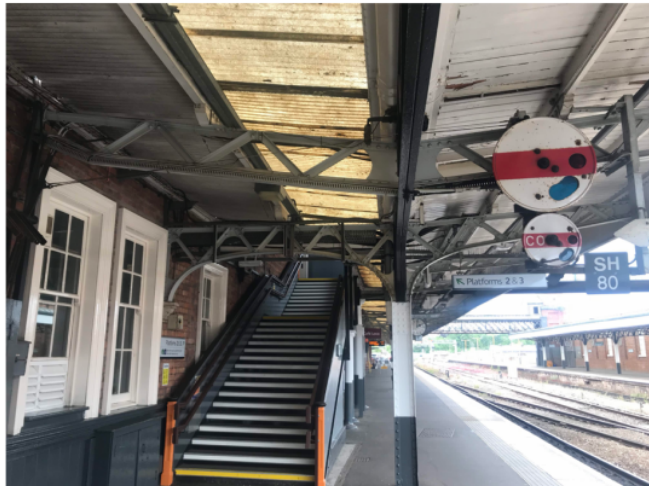
Figure 21 A Western Region round aspect banjo signal still in operational use on Platform 1 at Shrub Hill. Note that few layers of obsolete historic railway operational features are removed but are rather concealed.
