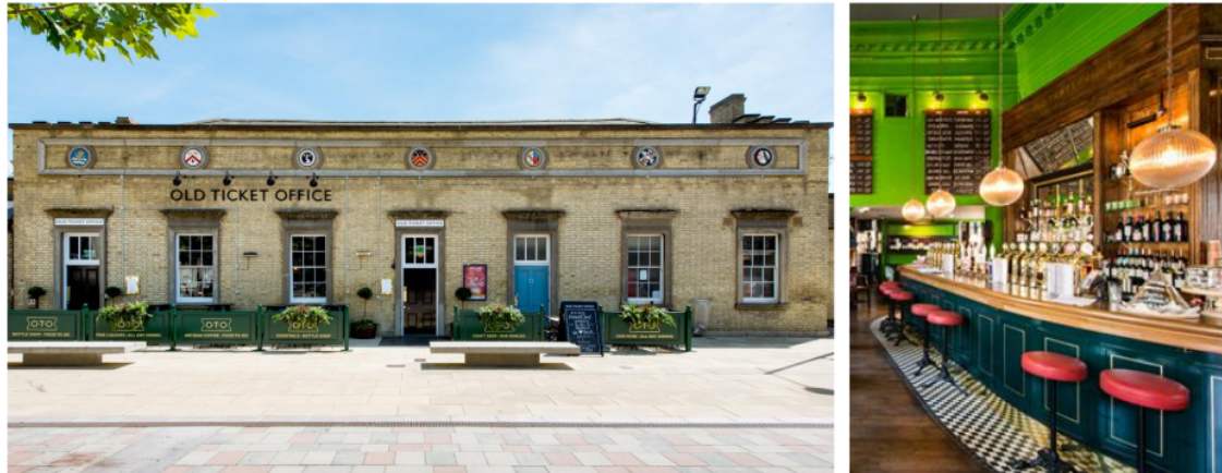
Figure 14 The new station pub situated within previously abandoned part of the station
