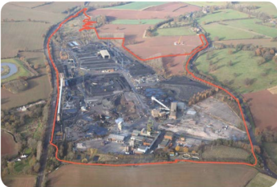
Figure 3.3. Mining site with physical facilities (Harworth Estates n.d.)
