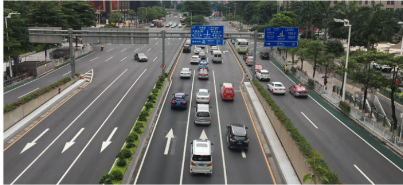
Fig. 5.6: Intersection of Huaxia Road.
