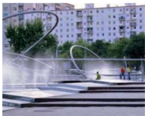
Figure 24. Mist generator (ibid)
