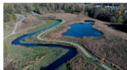
Figure 20. Constructed wetland (Ramboll, n.d.)
