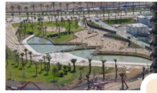
Figure 59. Diagonal mar park (Fluidra, 2017)
