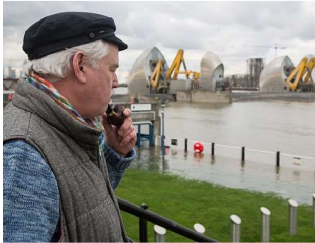
Figure 1. London flood issues in public open space (Telegraph.co.uk,n.d.)
