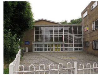
Lansbury Lawrence Primary School in the Lansbury Estate
