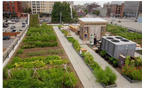
Figure 30 Food Roof Farm - first rooftop farm in St Louis situated at the heart of its dense urban core, roof is fitted with raised beds and other forms of growing
