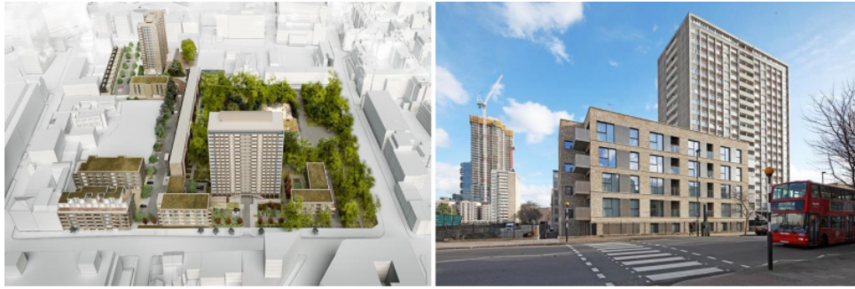
Figure 4.1 King Square Estate: plan and photo of new development (Pollard Thomas Edwards)
