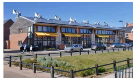
Figure 22. Sustainable housing with PV panels (Arup, 2010)
