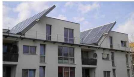
Figure 27. Housing with PV panels (Pizza Travel, 2014)
