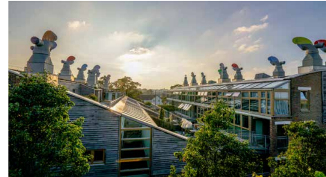
Figure 12. BedZED, South London (Zed Factory, 2009)
