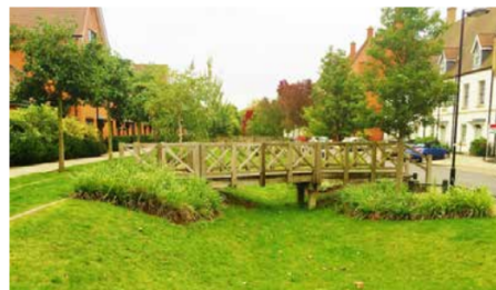
Figure 21. Vegetated bioswale (The Land Trust, 2015)
