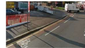
Figure 50: Narrow cycling lane on Hoe Street
