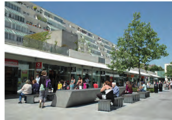
Fig 20: The active frontages of The Brunswick Centre ensure a good relationship with the wider street.
