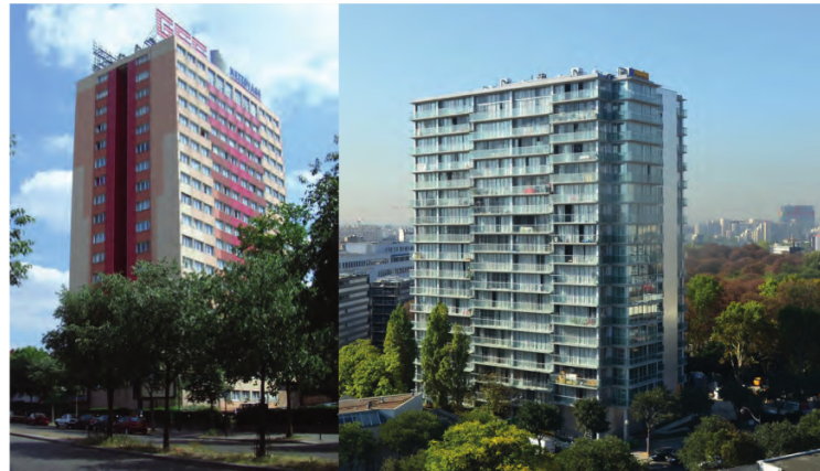
Fig 58: La Tour Bois-le-Prêtre, Paris. Before (left) and after (right) the retrofitting of balconies onto the social housing tower.
