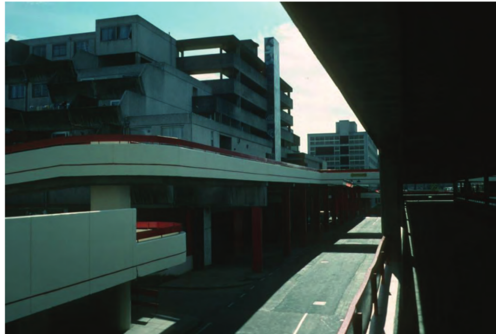
Fig 10: Walkways on the Broadwater Farm Estate, London, completed in the 1970s. High crime rates were seen in the areas beneath the walkways, as a result of the lack of overlooking and poor lighting. Many of the raised walkways have since been demolished, and along with other influencing social factors, crime rates have improved on the estate.
