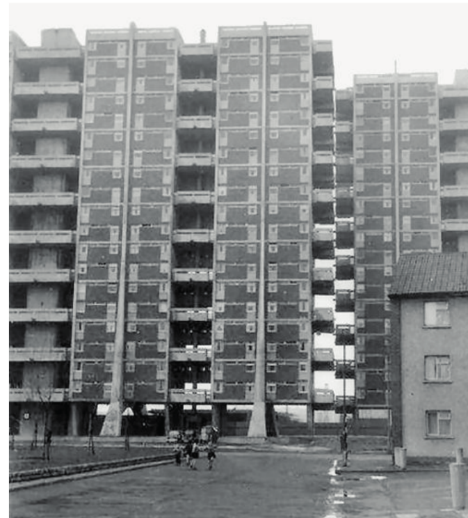
Fig 9: Hutchesontown C, Gorbals, Glasgow. Designed by Basil Spence, the development was inspired by Le Corbusier's masonette blocks in Marseilles, however failed to include any play space or facilities for children. The estate suffered from many other problems, including damp and infestation and was subsequently demolished in 1993.
