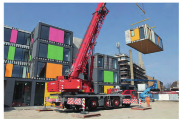
Fig 55: Speedy modular construction techniques are used.
