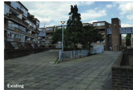
Fig 47: The existing podium is an area of hard-paved amenity space. Below the podium is garage space for cars.
