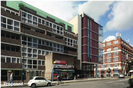
Fig 44: The eight-storey infill tower overlooks the street. It also provides active frontages at ground floor level and improves the estate's relationship with the street.
