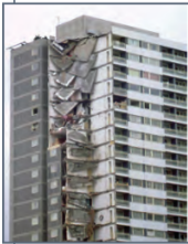
Fig 7: Ronan Point, built in 1968 collapsed 2 months later
