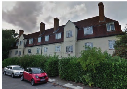
Slab block adjacent to site.
