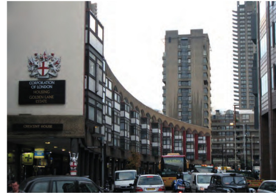
Fig 18: The active frontages of Crescent House ensure a good relationship with the wider street.
