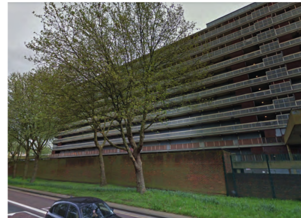
Fig 16: Haygate Estate. Image shows a poor relationship to the street.
