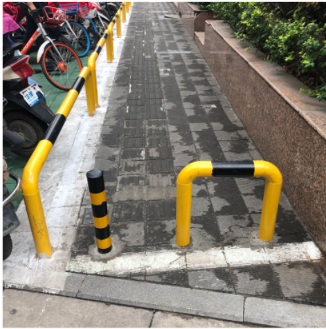
Figure 9, 10 and 11. Tactile paving impeded by other municipal facilities (Author, 2019).
