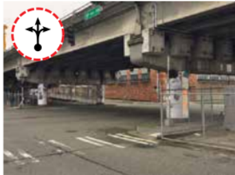
12.13 Underbridge with fences
