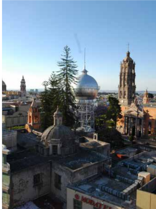
29.1 Water Tower, city centre, Celaya, Mexico
