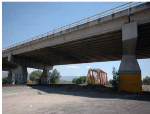
30.3 Line NB steel bridge & abutments, Celaya, Mexico
