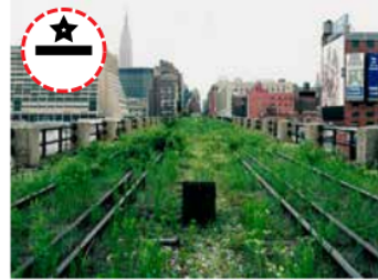
12.6 Above-ground viaduct, New York
