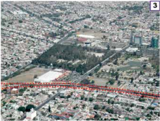
31.4 Line A, Xochipili I and II, south to north
