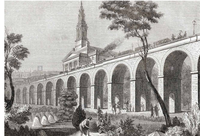
Greenwich Railway Viaduct, London c.1840 (Image: Transport for London Museum)
