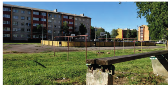
F34: Dilapidated courtyard space
