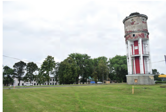
F42: 1950s water tower.
