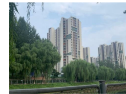
F51: Residential buildings under construction
