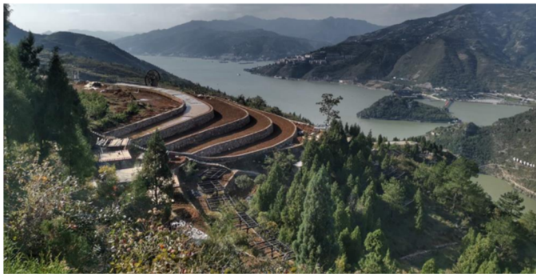
Figure 4.7. Construction of Terraces
