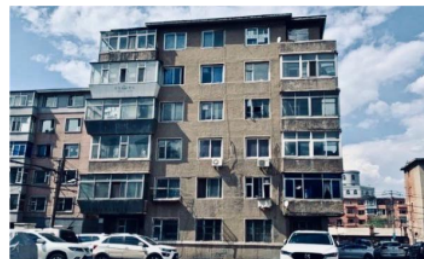
Figure 8 Old Residential Buildings (Source: Author, 2020)
