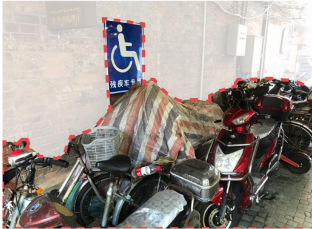
Figure 4. 1. 4: Parking space for handicapped cars is occupied by debris and motor bikes (Source: Author).
