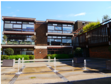
Figure 1.1 – the redevelopment incorporated brutalist architecture with high quality public-realm.
