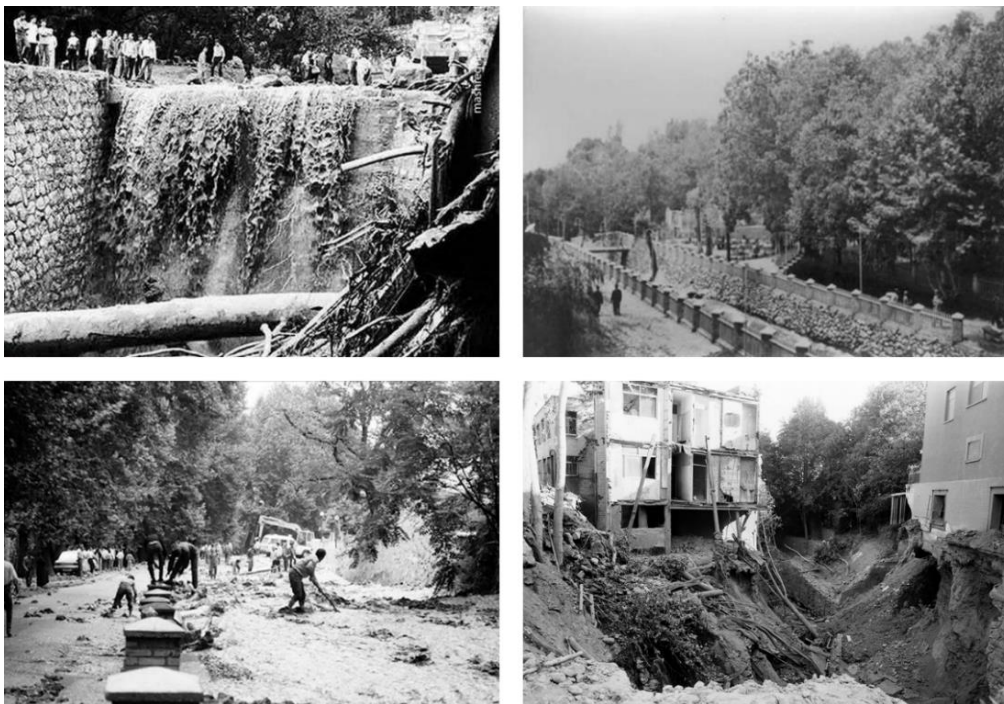
Figure 1.2 Darband river overflow (Up-Left), Darband river flood fortification (Up-Right), Tajrish Flood destructions (Down).
