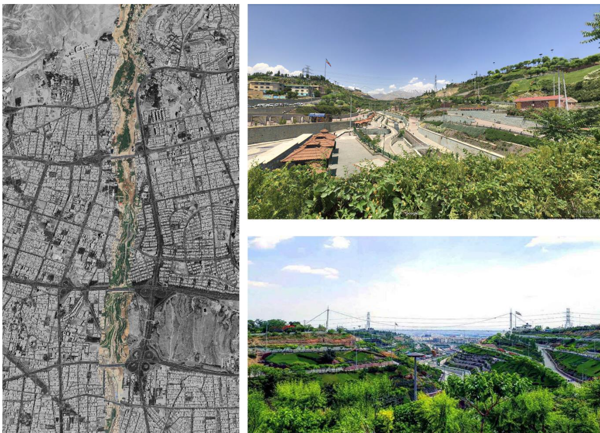
Figure 1.4 Farahzad river-valley (Left), Nahjol-Balagheh Park phase I (Right-up), Nahjol-Balagheh Park phase I (Right-down).
