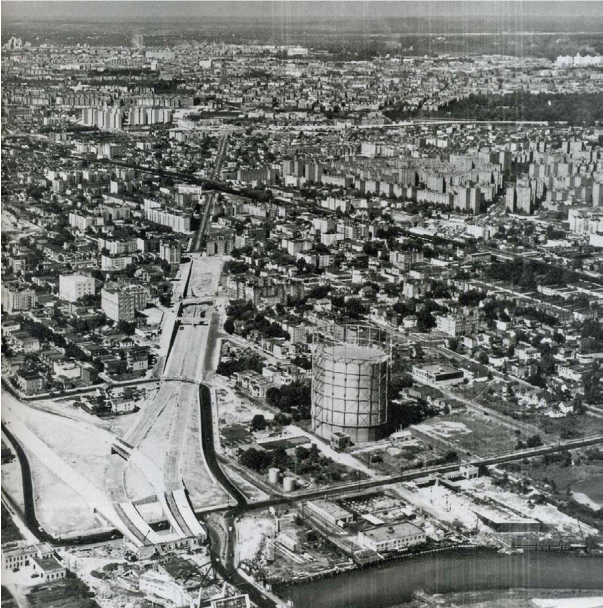
Figure 3 1950 construction progress of Cross-Bronx Expressway bisecting the street network Image source: 'Discovering NYC' Twitter
