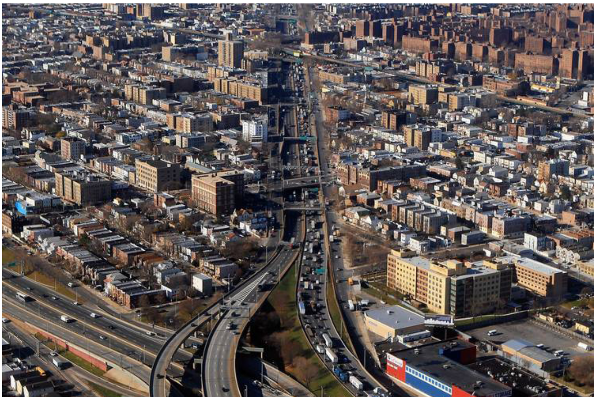
Figure 15 The Cross-Bronx Expressway from above showing trench condition, some streets are severed, others are continuous and bridge over
