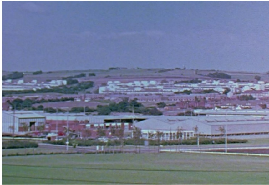
Figure 14: The new town from the south-west, 1971, with the Gillibrands industrial area in the foreground and the Tanhouse housing area behind. All the construction in this image had been undertaken since new town designation in 1961.
