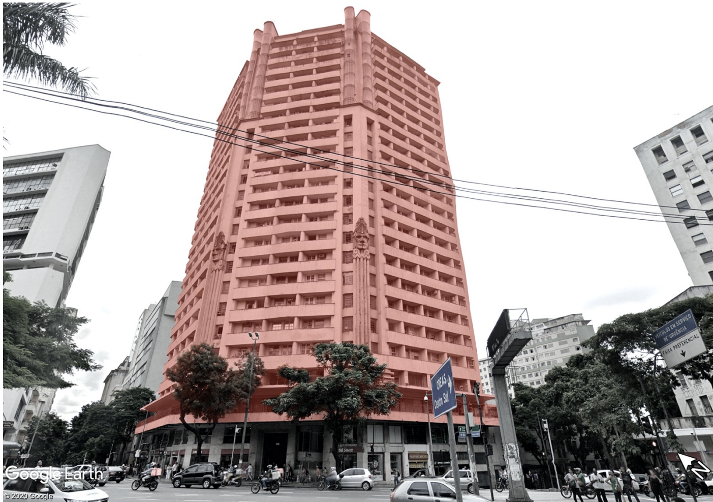
Figure 27: Area of interest 11 – Acaiaca Building.
