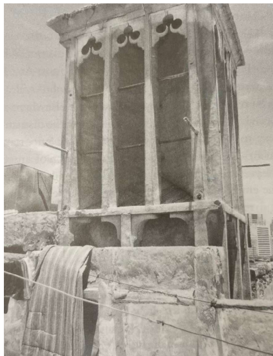
Figure 30: A Detoriating Wind Tower Used for Drying Clothes. Source: Dubai: Behind an Urban Spectacle
