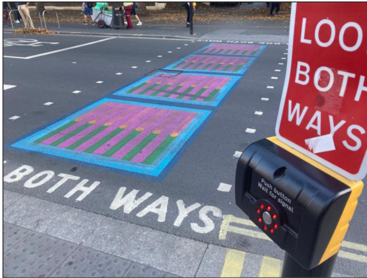
Photo.4 artistic designs add colour and interest to the street but are confusing to VIP that rely on standardised, recognisable elements to identify safe passage across roads
