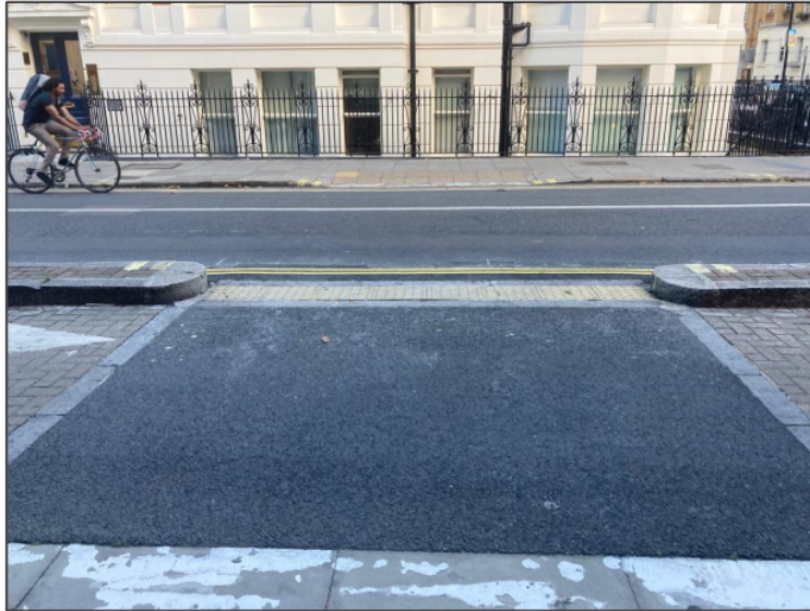
Photo.5 There are currently no signalling elements that inform VIP they are crossing a cycle lane
