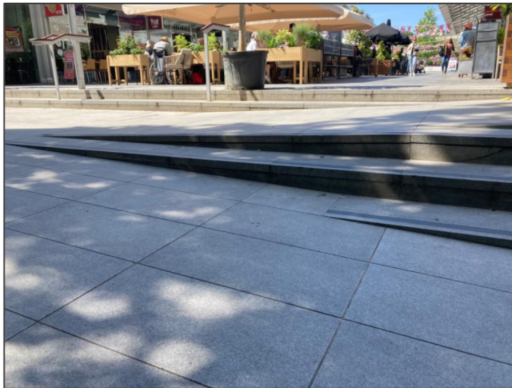
Photo.2 Inconsistency in the design of steps is anxiety producing and can be dangerous for VIP
