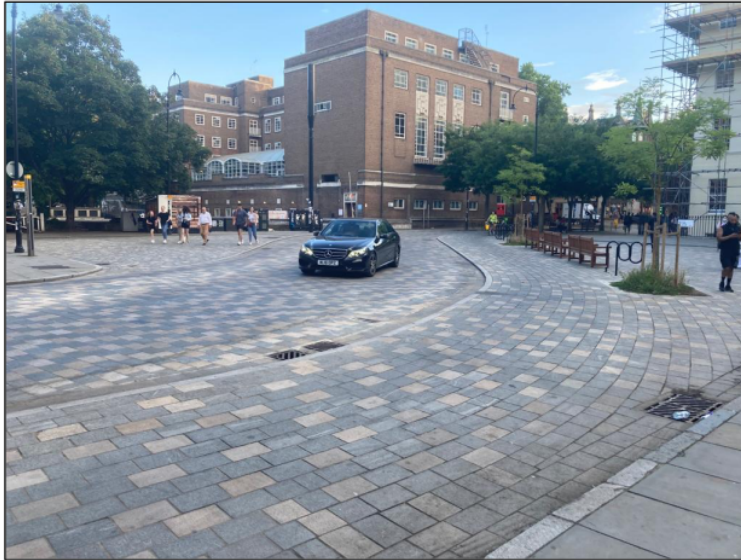
Photo.8 VIP are taught to navigate independently by following common elements of the streetscape. Removal of such elements renders the space inaccessible and potentially dangerous.
