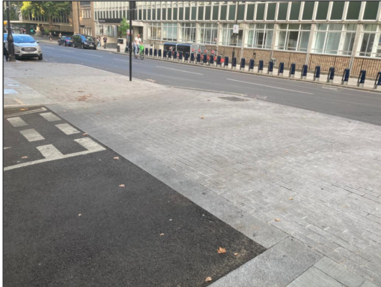
Photo.9 Continuous footways provide a false sense of security to pedestrians and exclude VIP through the removal of tactile markings
