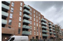
Newly-built mid-rise residential area
