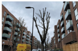
Newly-built mid-rise residential area
