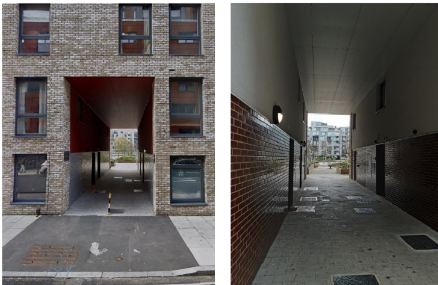
Figure 20: Views into the development from Wharf Road
