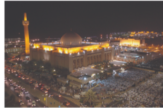
5 Fig 71: Grand mosque [listed building]
